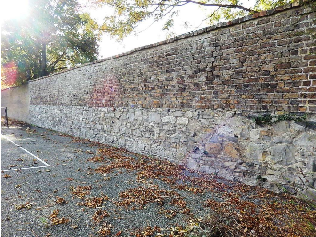
Rubble stone and brick garden wall to former wall garden now forms western boundary of tennis court.
