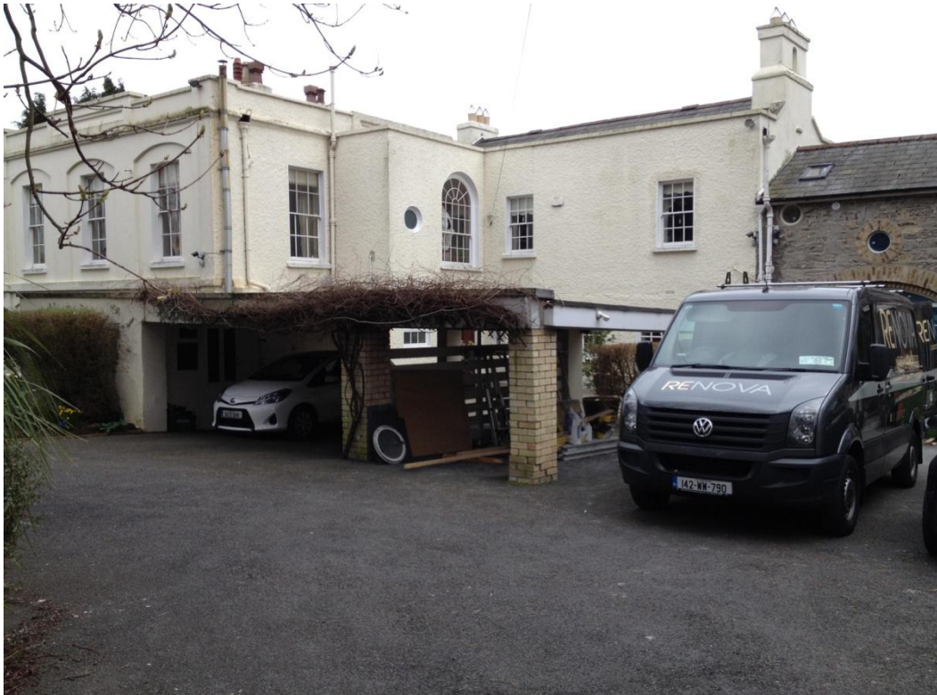
West-facing rear elevation of house with two-storey flat-roofed projection and north-facing elevation of the return. Former coach house with the stone elevation is located to the west (right of photo)
