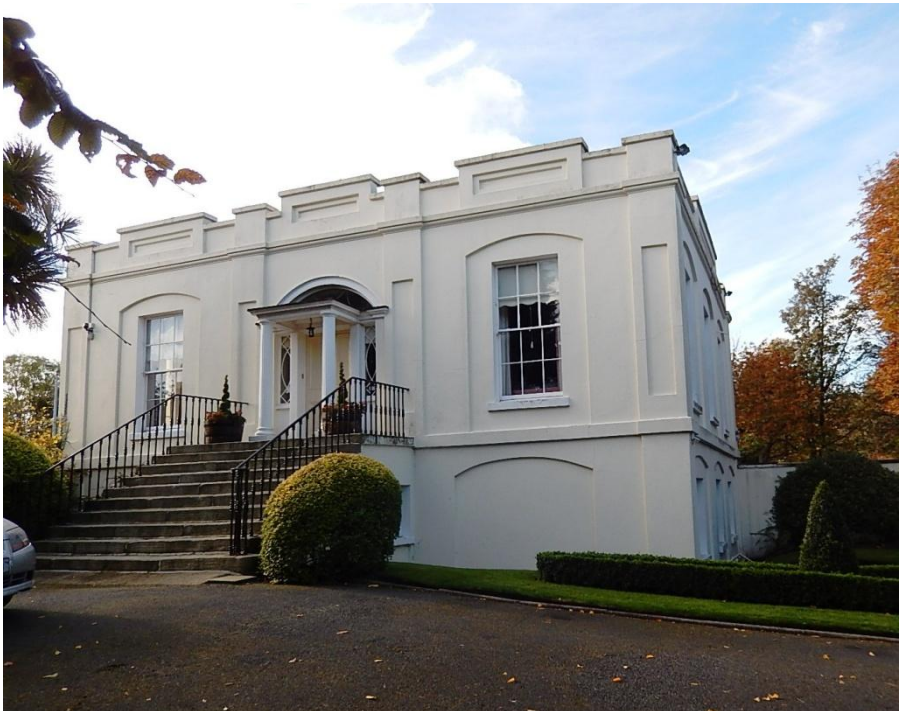
Front east-facing elevation with formal entrance steps
